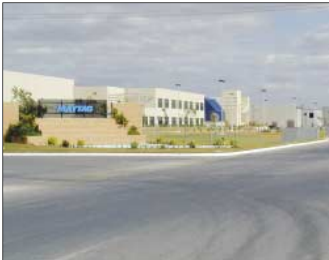
This Maytag maquiladora was recently built in Reynosa, Mexico. (Photo courtesy of Chad Broughton.)
